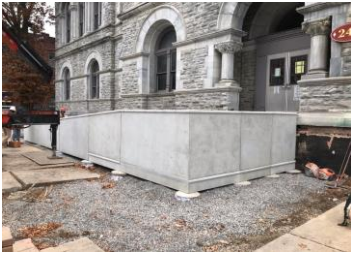
Ramp at Main Entrance of City Hall
